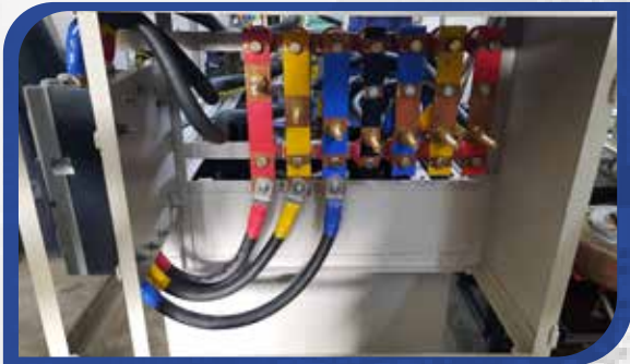
INTERNAL SECTION OF SERVO CONTROL VOLTAGE STABILIZER
